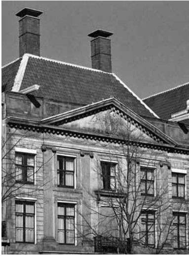
Herengracht 527 Cornice-gable with triangular pediment
